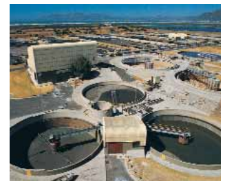
Ozone is being increasingly used as a disinfectant in water treatment plants
